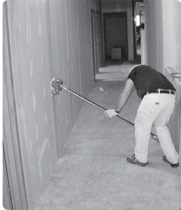
Problem: Hand drywall finishing with mudbox
