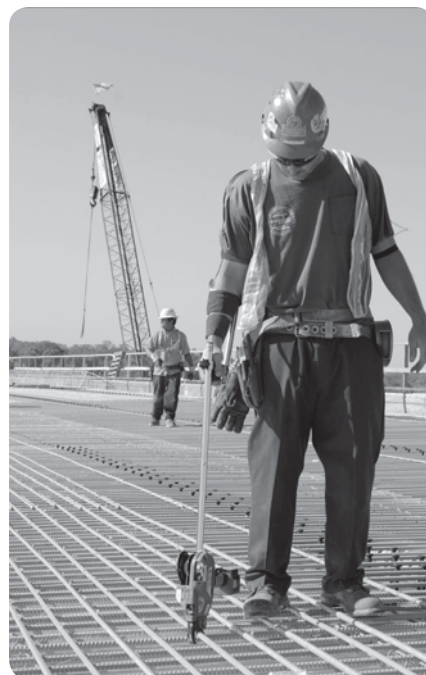
Solution: Rebar-tying tool with extension handle
