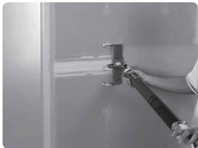
Solution: Pneumatic finishing system
