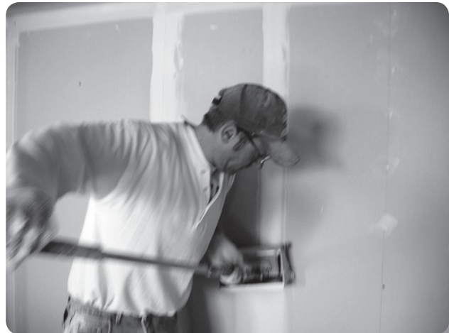
Problem: Hand drywall finishing with mudbox
