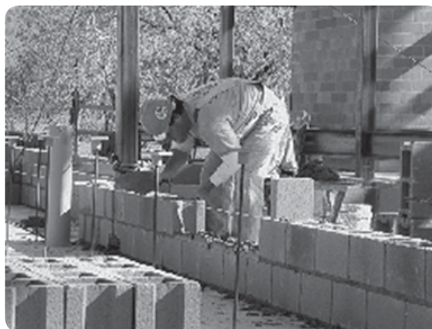
Problem: Laying standard concrete block
