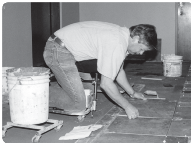
Solution: Laying tile with kneeling creeper
