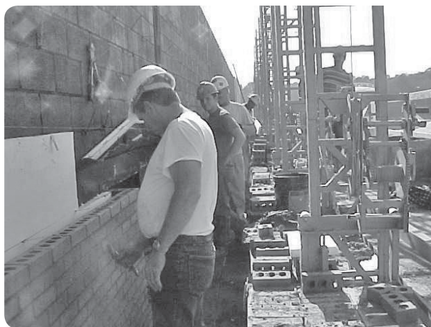
Solution: Masons finish top course on split-level adjustable scaffolding
