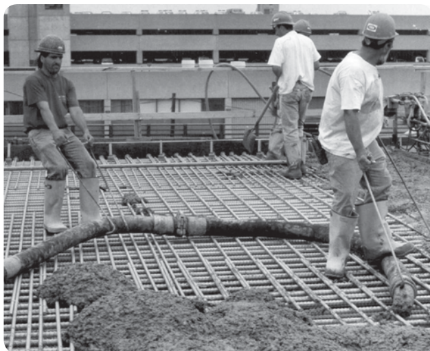
Problem: Pulling concrete hose without skid plate
