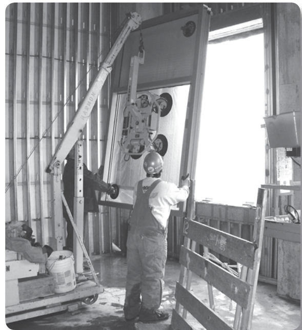
Power vacuum lifter avoids manual lifting
